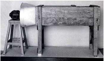
Figure 2: The Wright wind tunnel [9].
